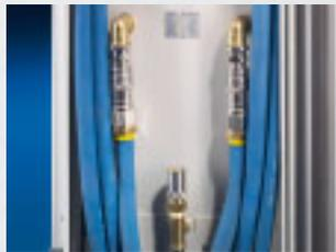
Fasteners. Splash-free quick-release fasteners facilitate retrofitting and maintenance of individual modules while the system is operational.
